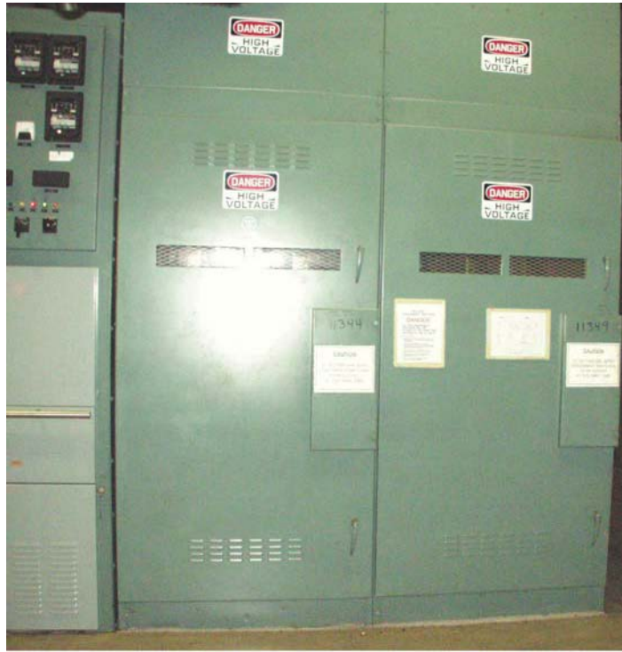
Fig. 1 WESTINGHOUSE 34.5KV LOAD INTERRUPTER SWITCH TYPE WLI
